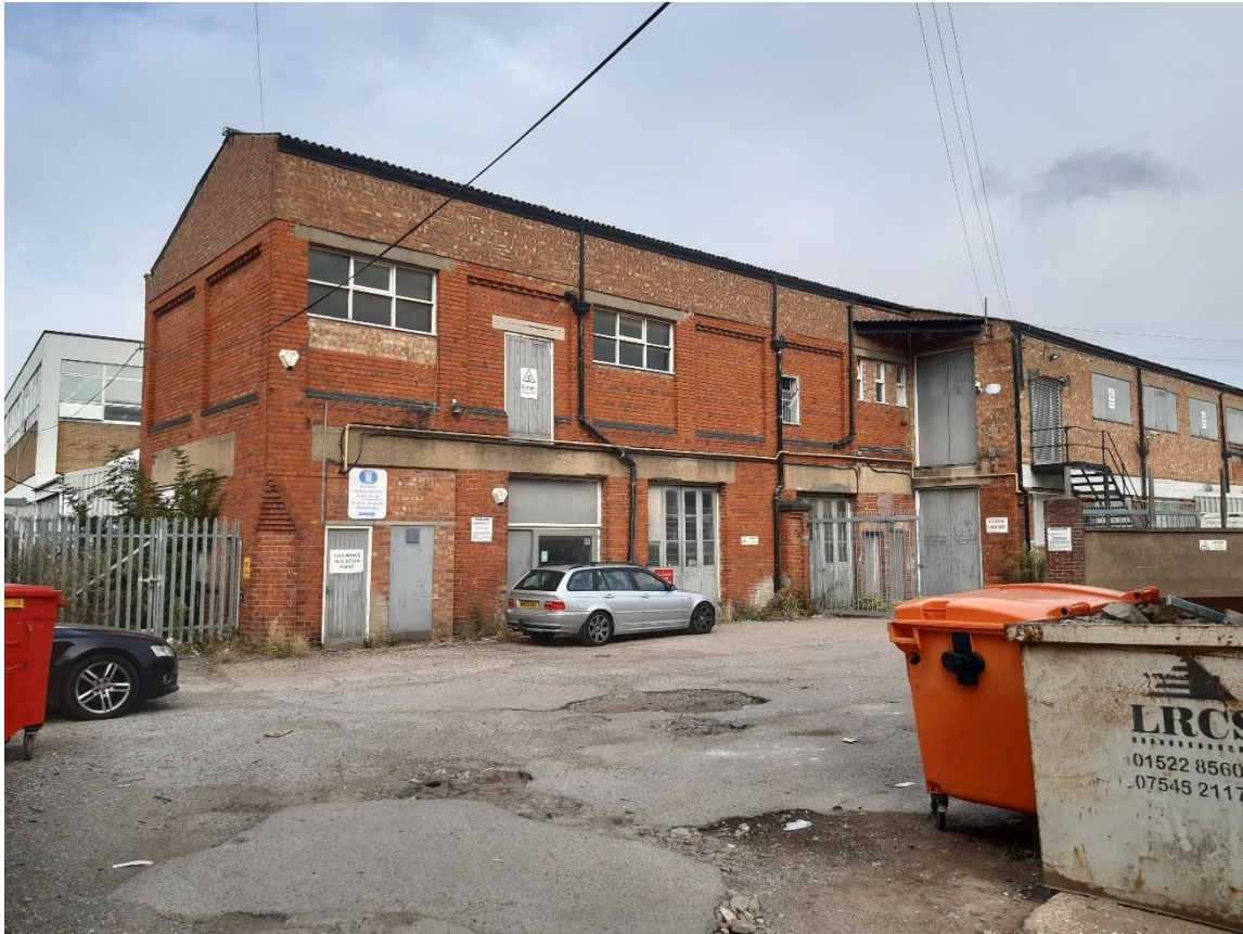
Existing warehouse with Royal Mail Sorting Office behind
