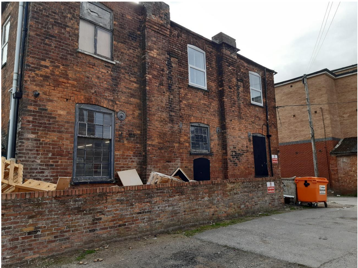
Rear elevation of 134 High Street
